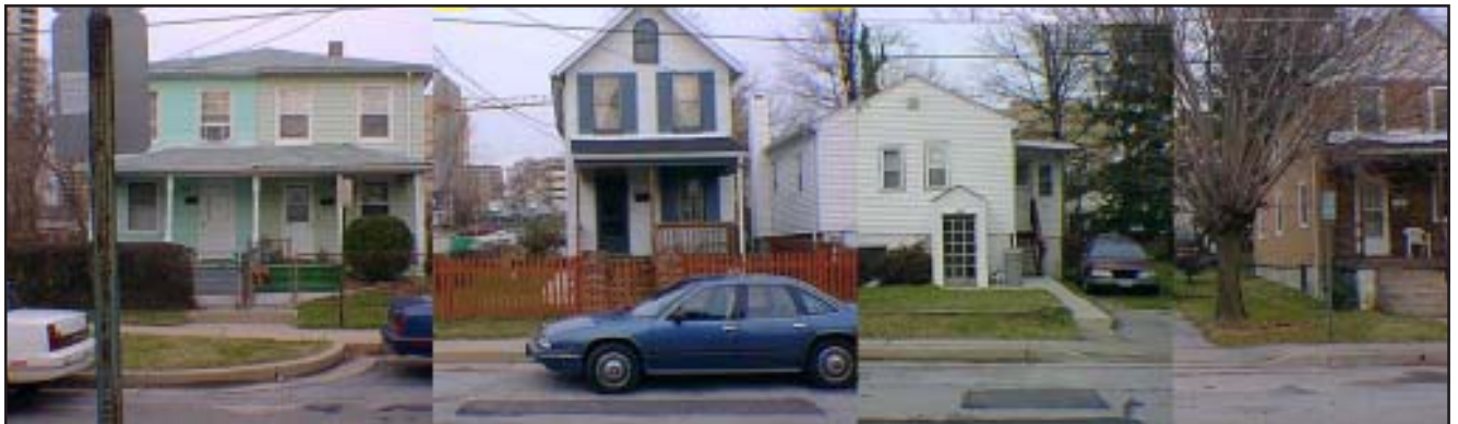
A mix of housing shapes and side setbacks on Lennox Avenue produces a varied building rhythm.
