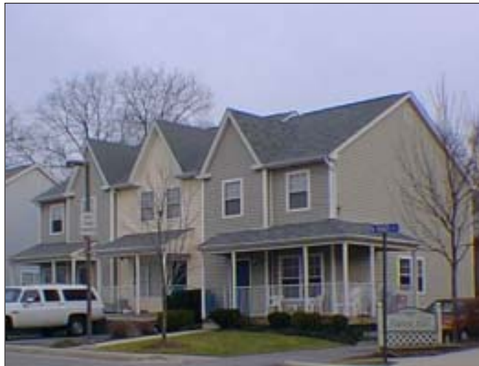
This multifamily construction in East Towson used gables on the front facade, front porches which wrap around the building at the corners, and compatible materials and colors to blend in with the historic architecture.
