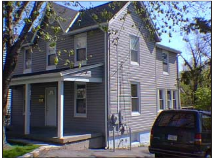
Using wall and roof offsets provide an effective method of minimizing color and material differences and provide a complementing transition between the old and new.
